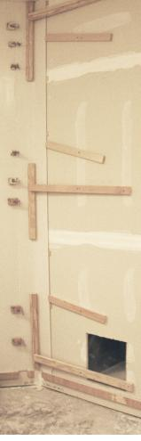
Use vacuum clamps and/or bracing to pull or push and hold seams together. Adjustment blocks can be mounted with hot melt glue to help align adjacent surfaces to achieve inconspicuous seams. Use of a wooden shim is shown in top right view to maintain silicone adherent thickness. Figure P-2 shows the assembly of a tongue and groove seam for 6 mm (1/4") solid surface sheet.
