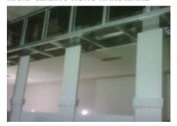
Each Privacy Plus® pilaster is manufactured with a metal plate built into the top. This is built into the solid surface material in such a way that it can not slip out. The plate is then bolted into a steel C-Beam in the ceiling for support and strength. Once the plate of the pilaster is bolted in, the pilaster will not move even when pushing against it.
