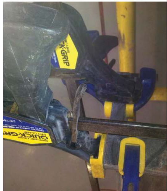
Figure F-8: Clamping left end cap backsplash segment
