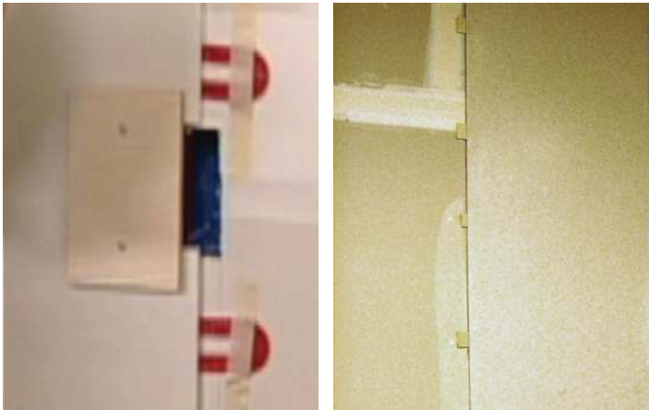
FIGURE A-2: SHIMS MAINTAIN MINIMUM SILICONE BOND LINE THICKNESS (SHIMS CAN BE SECURED WITH HOT MELT GLUE AND LEFT IN PLACE)
