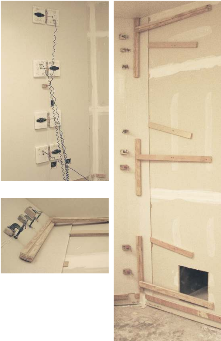
FIGURE P-1: CLAMPING SEAMS
