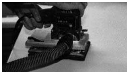
Buff the surface with a Scotch-Brite® pad.
