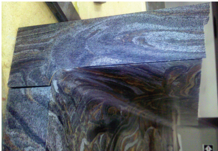
Figure F-7: Left end cap, backsplash portion dry fit
