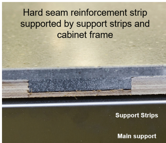
Figure M-4: Hard Seam Reinforcement and Support
